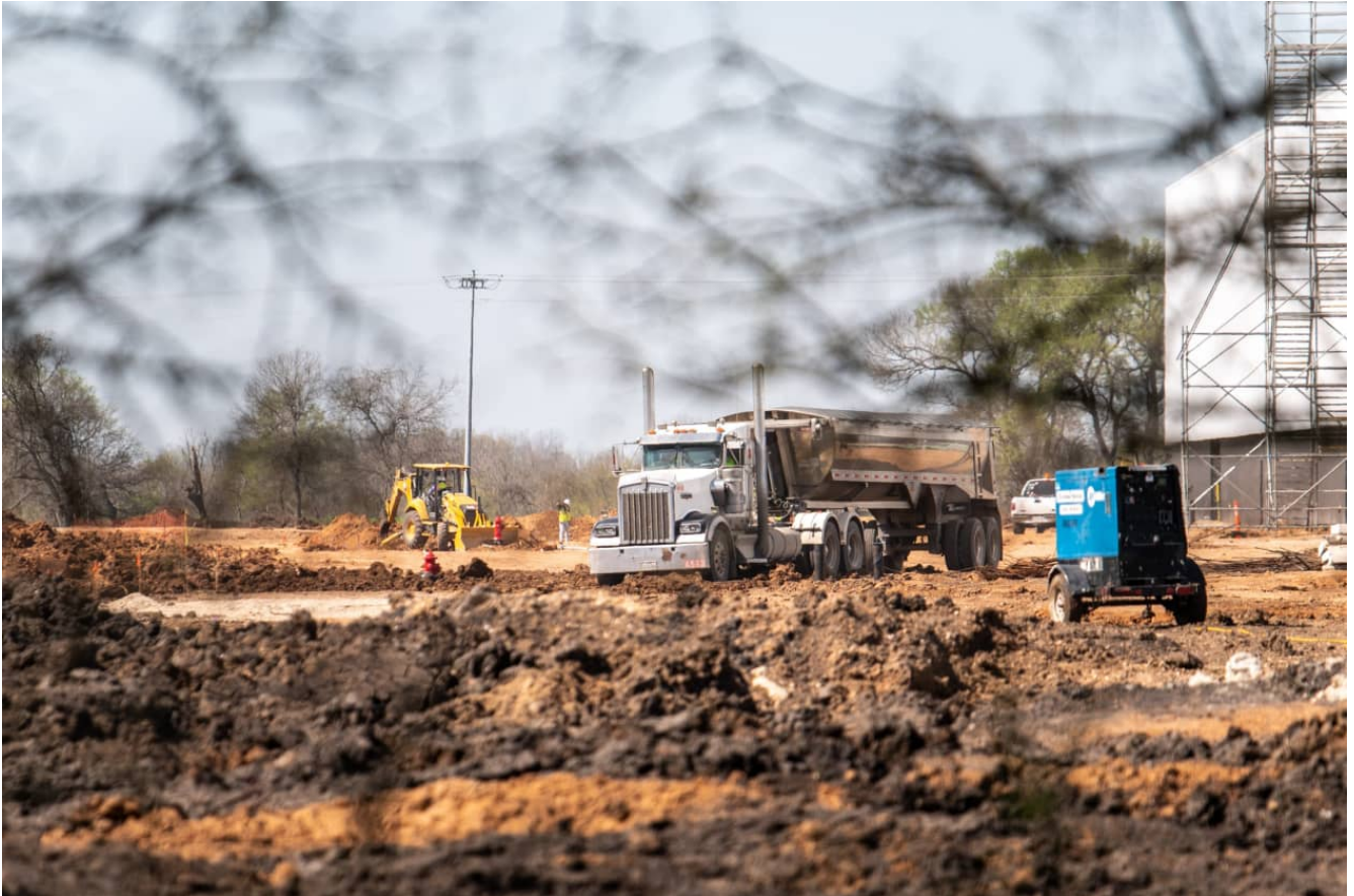
Construction at a SpaceX site in Bastrop County in February.
